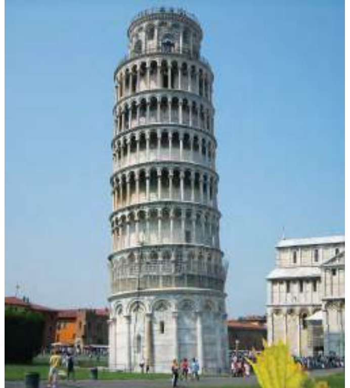
Leaning Tower of Pisa
